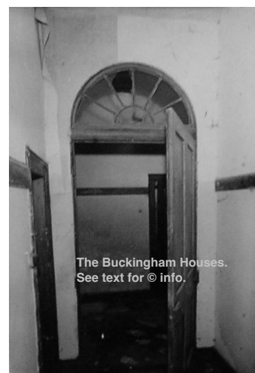
7. Service passage looking east
