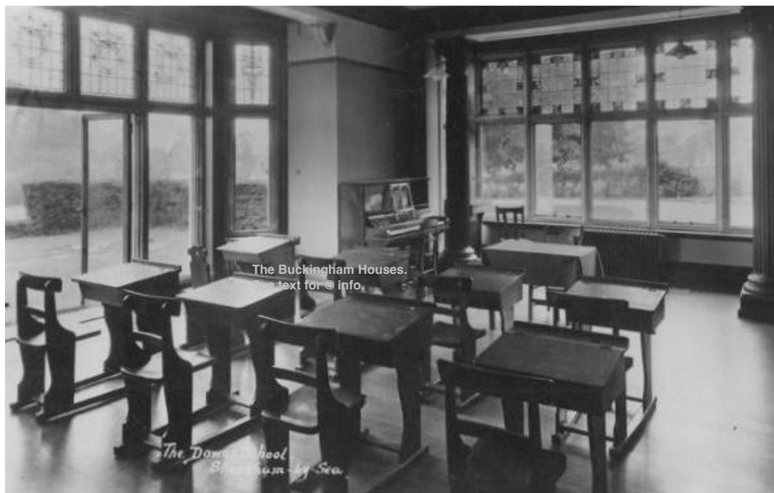
Classroom on ground floor of southwest corner
