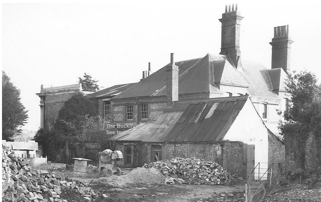
North elevation from Ravensbourne Avenue
