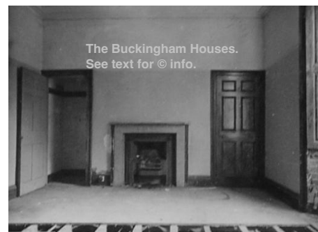
8. Northwest bedroom looking west
