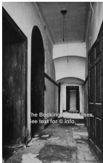
6. View north to billiard room
