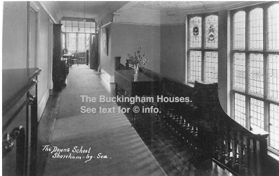
Landing and top of main staircase
