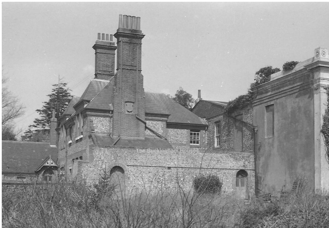
West and south elevations
