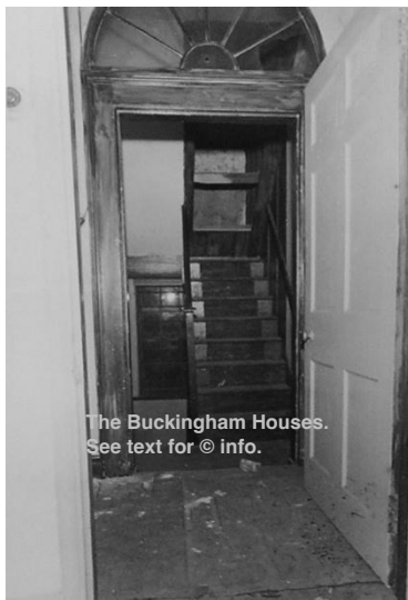
5. Stairs looking north
