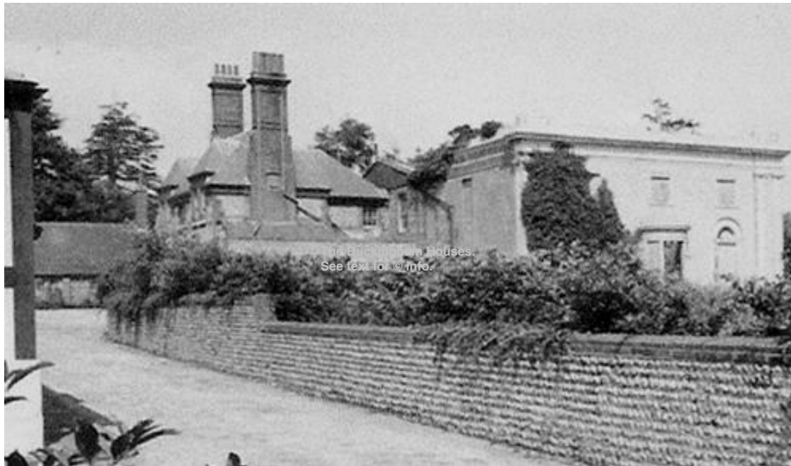
West and south elevations from Buckingham Mews
