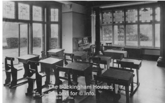
Classroom on ground floor of southwest corner
