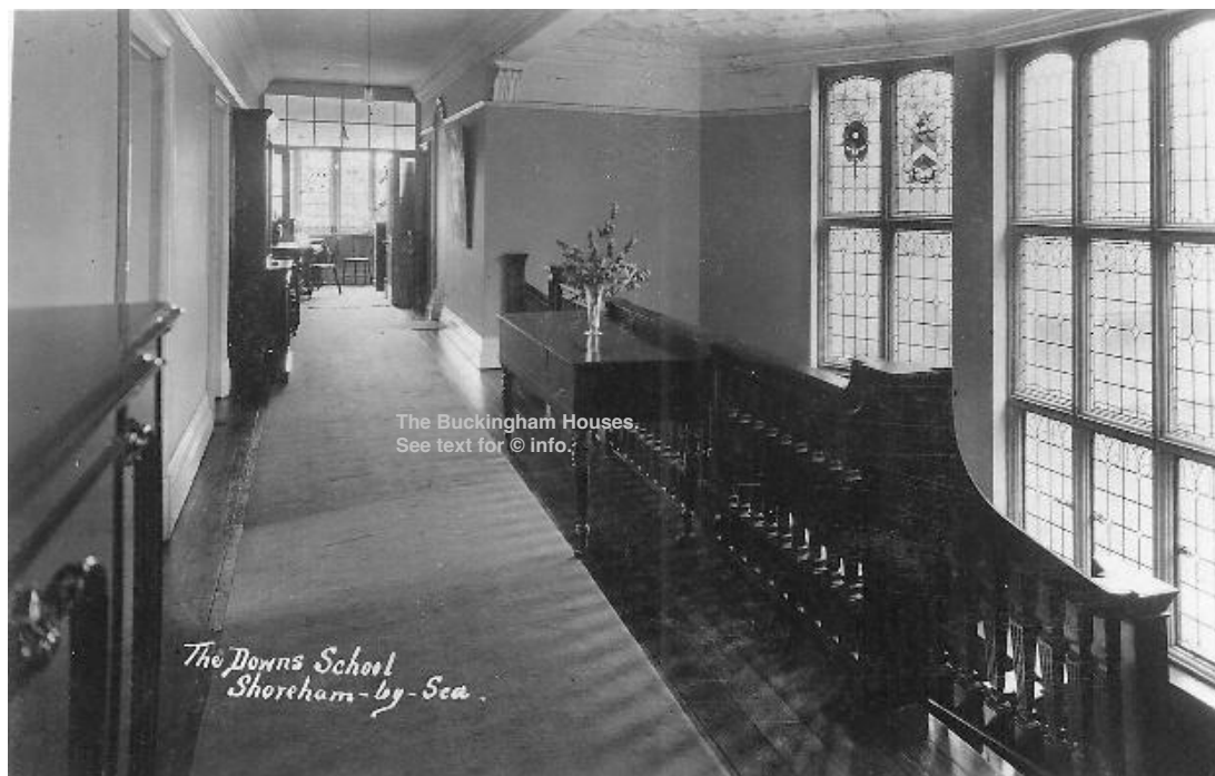
Landing and top of main staircase
