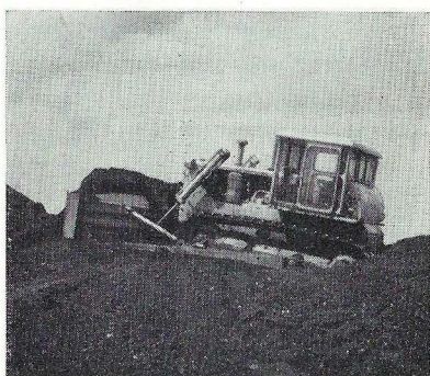
Some coal goes to a reserve stock-pile and is consolidated by bull-dozers to prevent spontaneous combustion.
