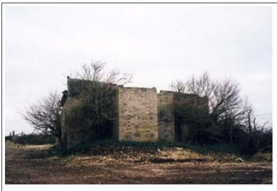
The remains of T2 transmitter block blast wall in 2007.
