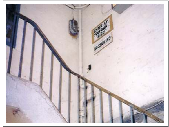
The stairs at the back of the guardroom lead down to the tunnel. (Howard Toon)
