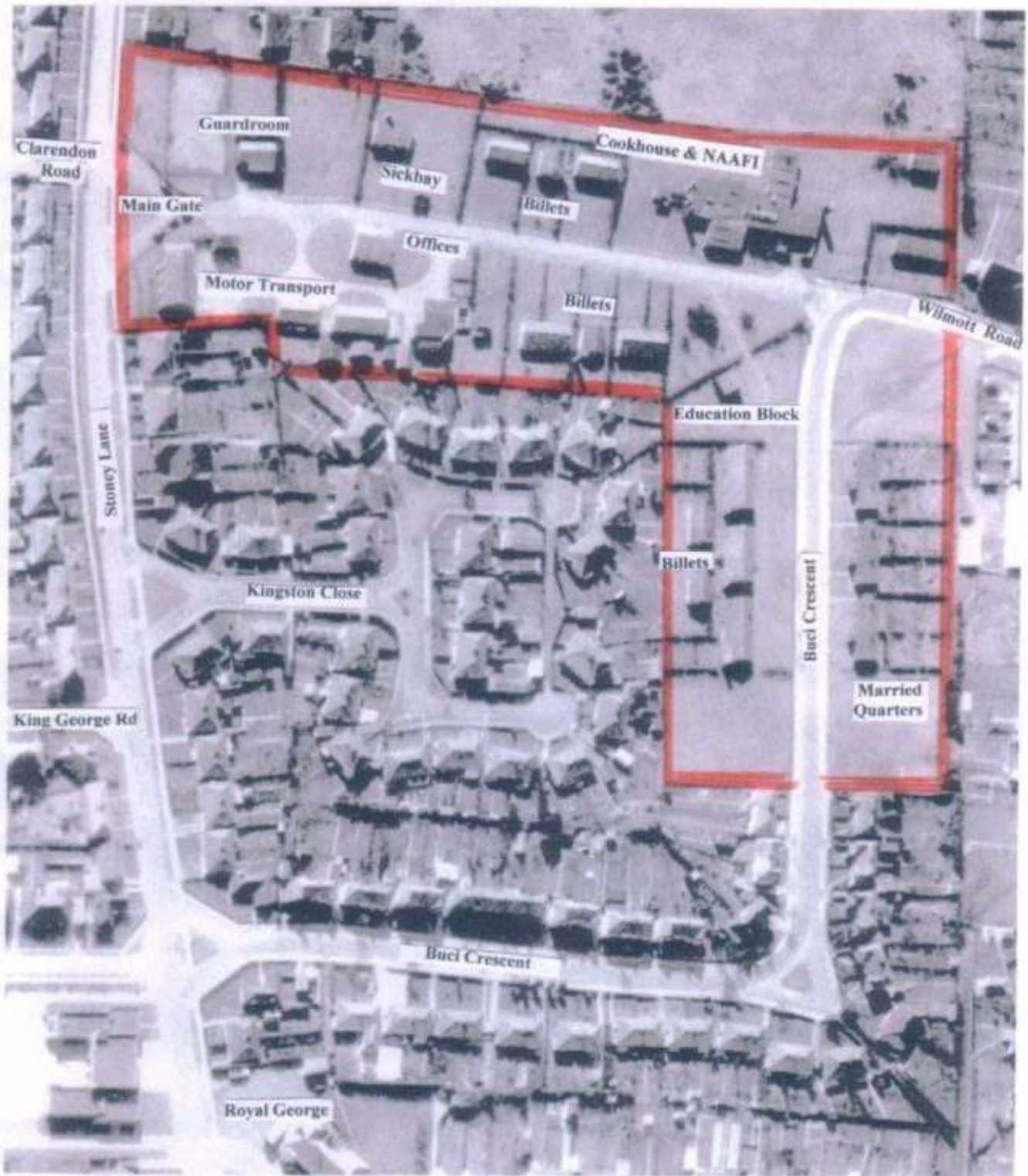
Aerial view of the Truleigh Hill domestic site shortly before demolition in 1965. (West Sussex Records Office)
