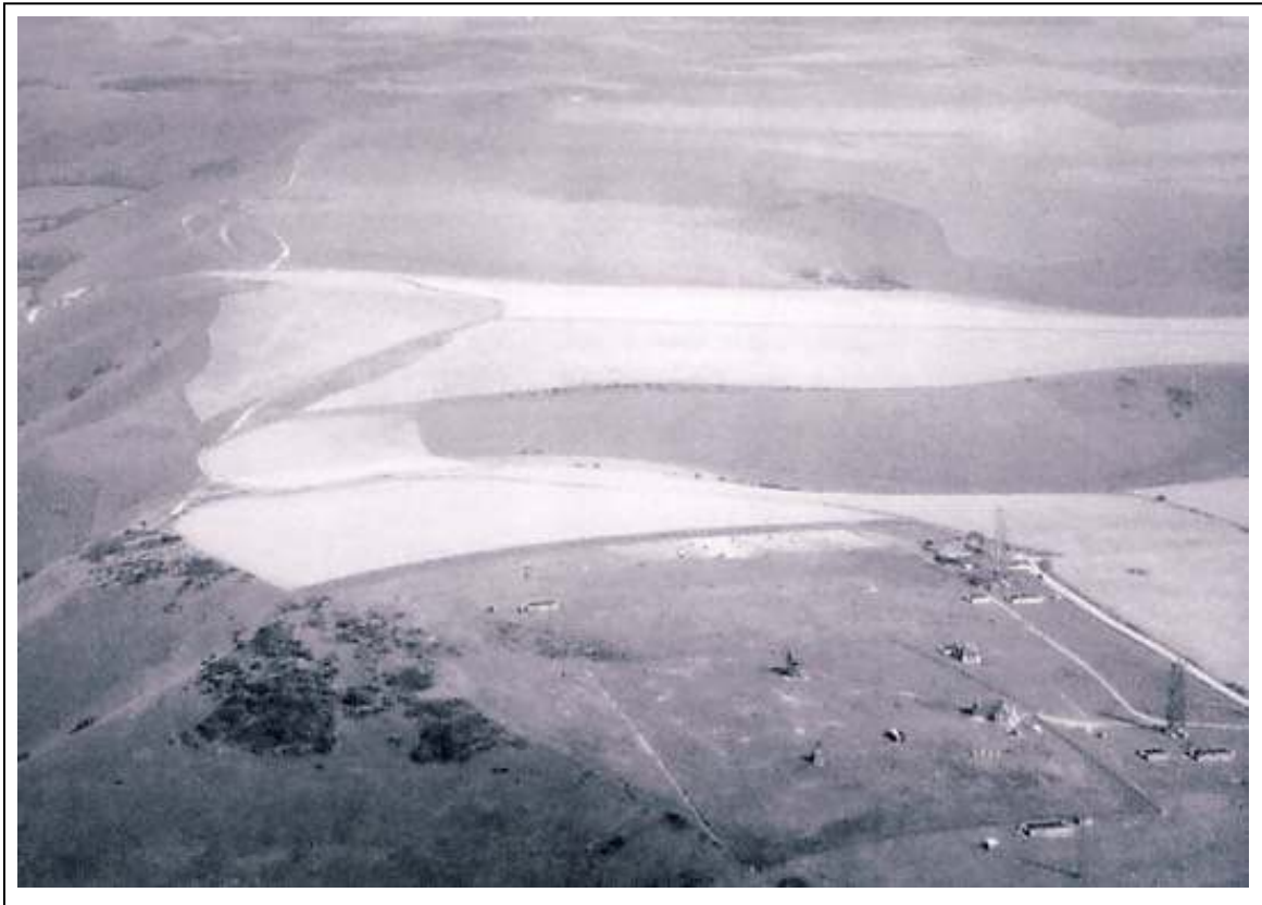
Two views of the technical site taken in 1954-55. The lower view shows the present South Downs Way heading across to Devils Dyke at the top left hand corner of the picture. (RAF Museum, Hendon)
